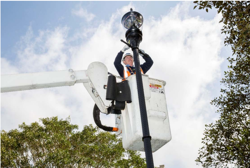
Left: installing LED lighting at Hollis Park.
