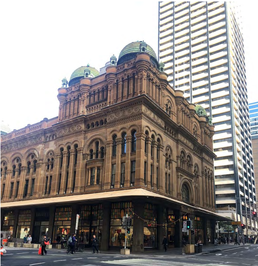
Figure 2 – The Queen Victoria Building as viewed from corner of George and Market Streets
