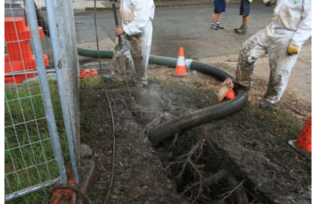
Figure 95- Hand excavation or other non-destructive methods such as water jetting and vacuum extraction to excavate around tree roots. (Photo: Arterra)
