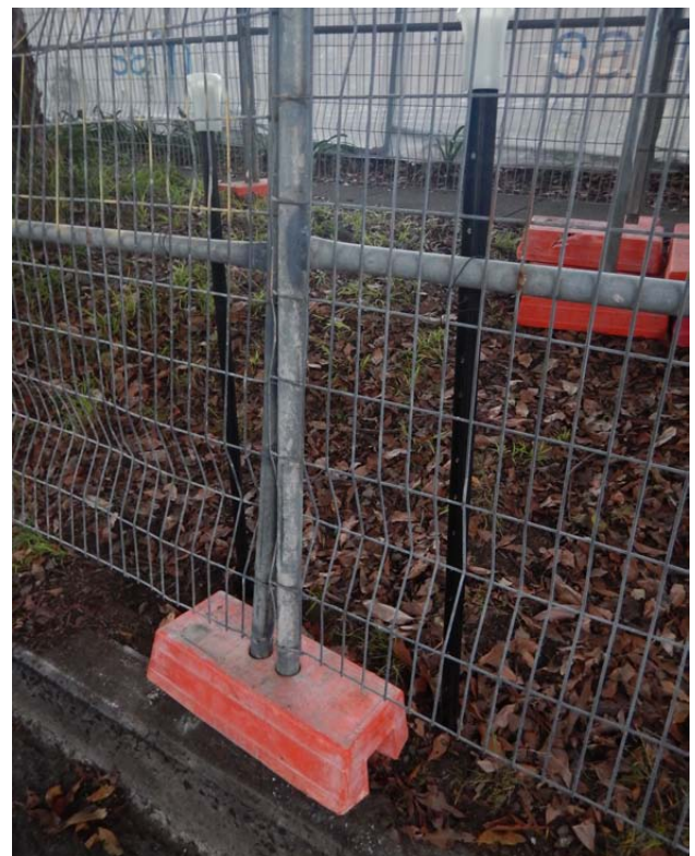
Figure 92- Where ground is uneven or the site is subject to strong winds the fencing may be held securely by wiring to strategically placed star pickets driven into the ground. (Photo: Arterra)
