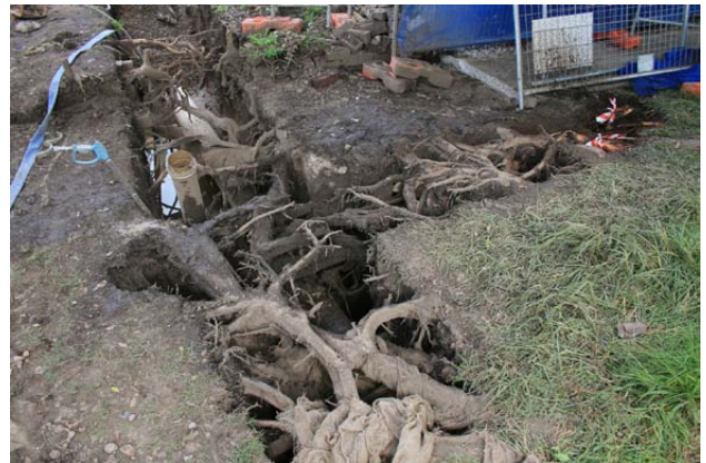
Figure 96- Non-destructive excavation methods can allow services to be installed across verges without the need to sever important and structural tree roots. (Photo: Arterra)
