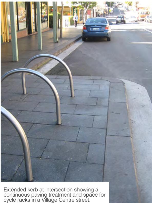
Extended kerb at intersection showing a continuous paving treatment and space for cycle racks in a Village Centre street.
