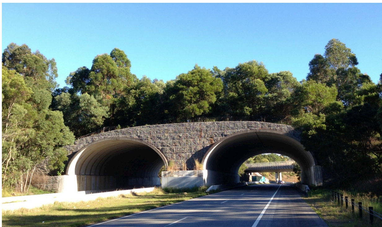
Example of vegetated fauna overpasses in northern NSW. While overpasses of this extent may not be feasible at St Peters, smaller versions could potentially be incorporated with proposed cycle/pedestrian bridges.
