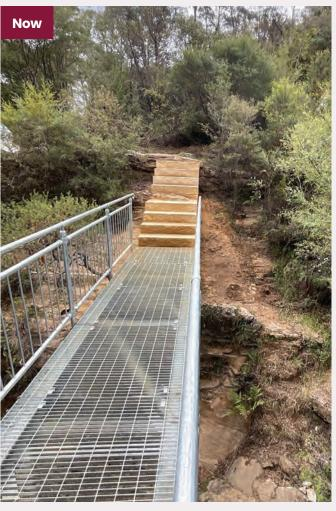
It was clear that more resilient infrastructure was required. A new track alignment was established away from the creek. Resilient design elements included replacing timber steps with sandstone, and installing steel footbridges and elevated boardwalks using techniques that minimised disturbance to the environment.
