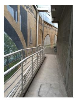
Ramp to level 1 is 1010mm wide and includes continuous handrails on the right-hand side.
