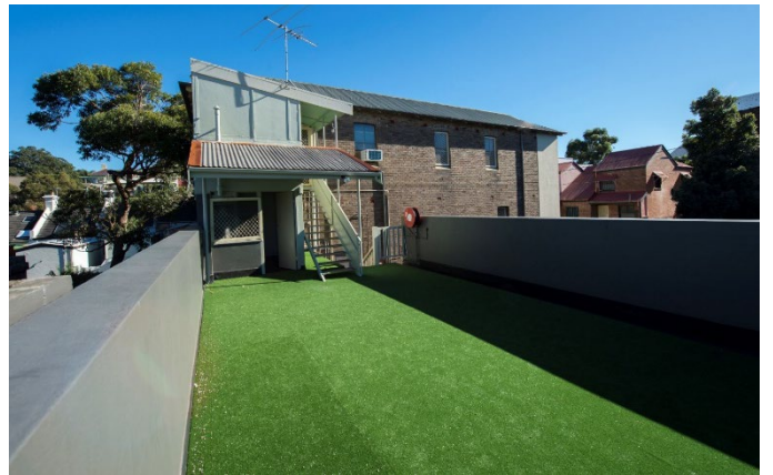
Image: view across terrace to laundry of Waterloo Creative Live/Work Space.
