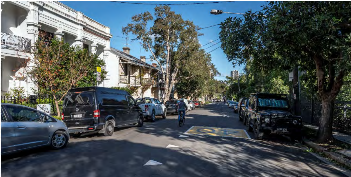
Figure 3-6 Previous configuration of Bridge Street (looking south)
