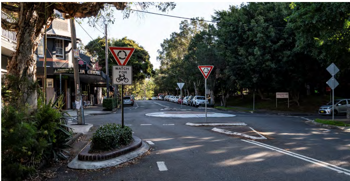
Figure 3-8 Previous configuration of Henderson Road (looking west toward Alexandra Street roundabout)
