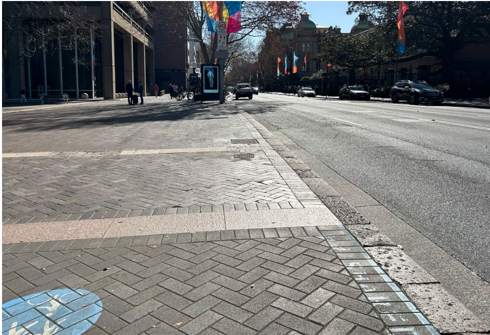
Figure 6-2: Mix of trachyte and concrete kerb, western kerb of Macquarie Street (AECOM, 2023)
