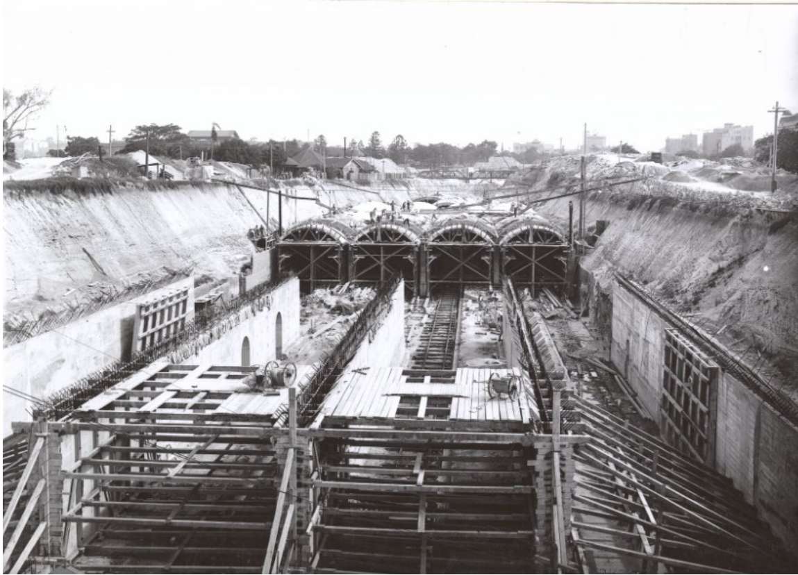
Figure 3-20: Excavation for the construction of tunnels and station, City Circle, St James NSW, c.1922. Note the four tunnels (Source: NSW State Archives & Records, Item NRS-17420-2-27-855/103)
