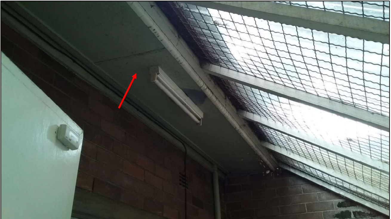
Photo 3: Interior, kitchen, eaves exterior panels (extends through kitchen above cupboards) containing asbestos
