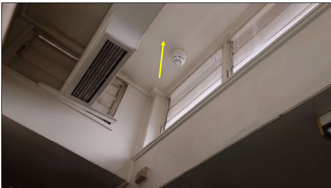
Photo 2: Interior, kitchen, ceiling panels, lead based white paint system
