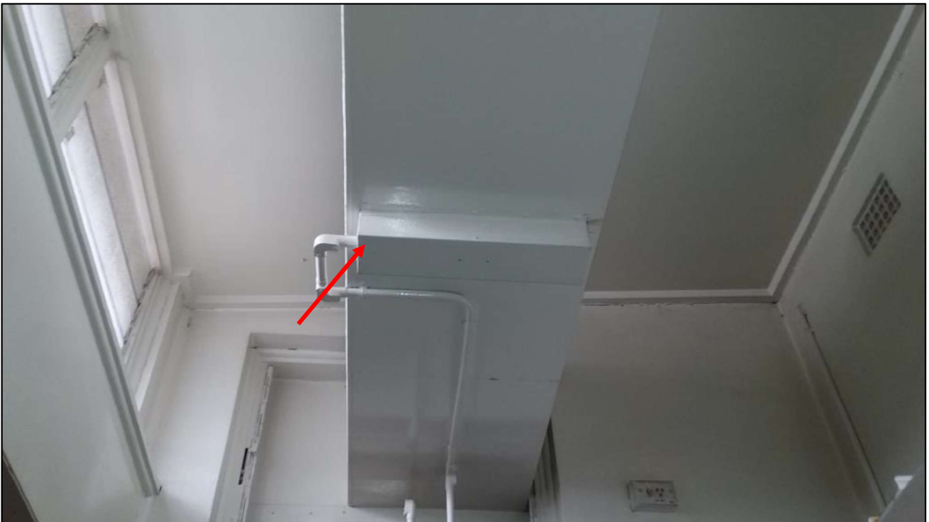
Photo 4: Interior, kitchen, vents, electrical duct heating with asbestos presumed present
