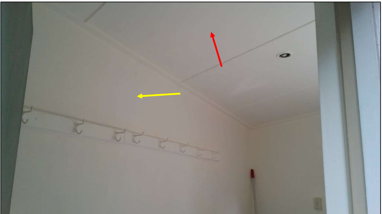
Photo 6: Interior, laundry and bathroom building, ceiling, fibre cement sheeting containing asbestos and walls with white paint system containing lead
