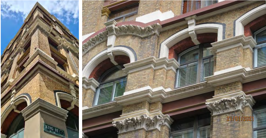
3 Exterior detailing to Broughton House. Source: TKD Architects, 2021.
