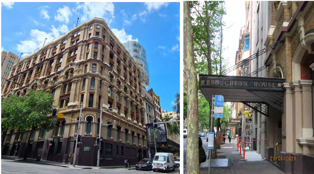
2 Broughton Hall as seen at corner of King and Kent Streets (L), and Broughton House awning and entrance on Clarence Street (R).
