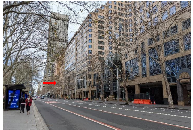
Figure 4 – Looking south along Elizabeth Street.
