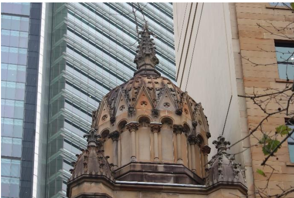
Figure 18 – Detail of sandstone tower dome.
