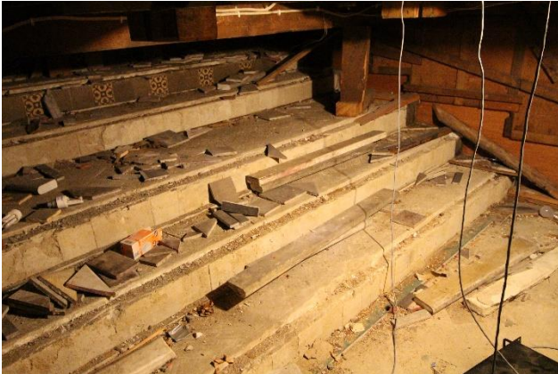
Figure 40 – Original stairs to Ark located under bimah.
