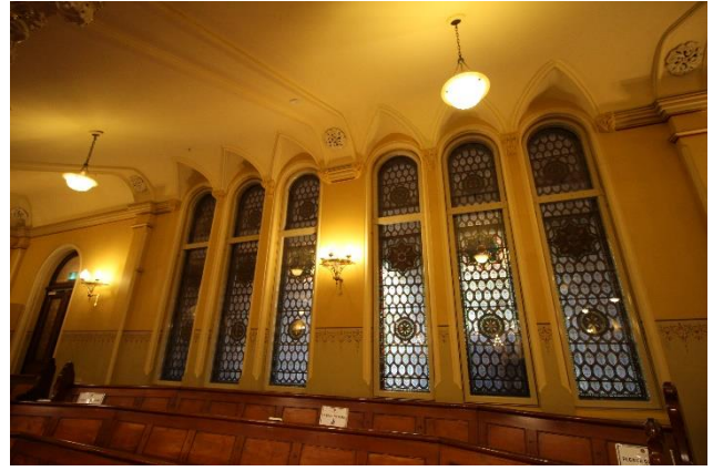
Figure 37 – Leadlight windows in Mens Gallery to porch.
