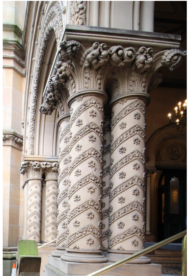
Figure 21 – Detail of columns to portico.
