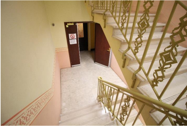
Figure 54 – Fire stairs in Education Centre.
