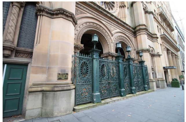
Figure 19 – Ground level at Elizabeth Street with original iron gates.
