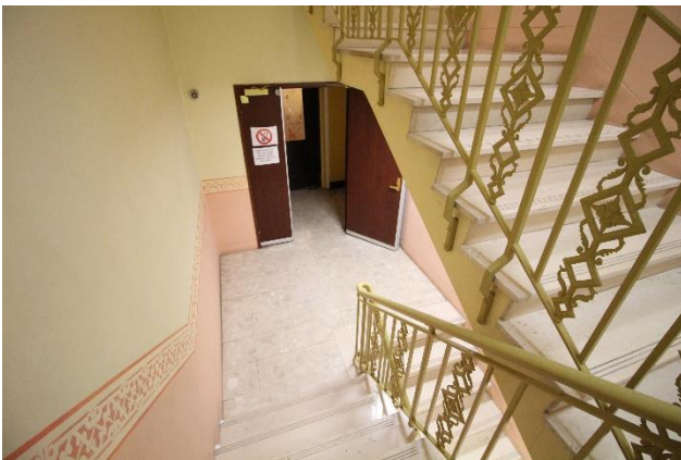
Figure 43 – Fire stairs in Education Centre.
