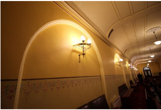
Figure 19 – Wall mounted gasoliers in Ladies Gallery.
