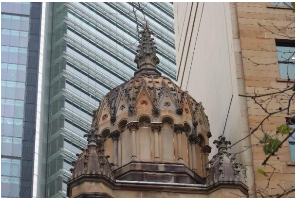
Figure 7 – Detail of sandstone tower dome.
