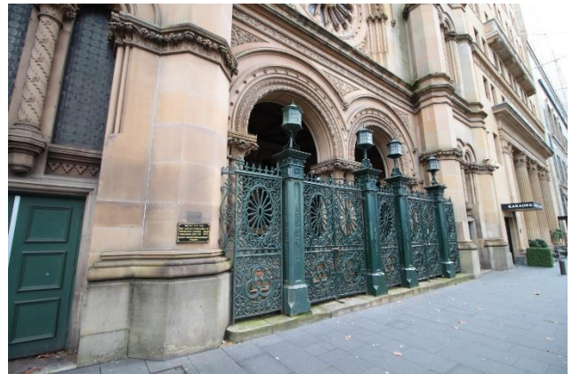
Figure 8 – Ground level at Elizabeth Street with original iron gates.
