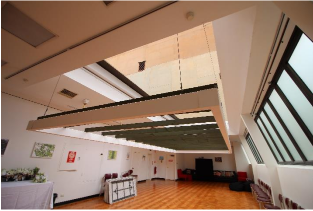
Figure 41 – Succah with roof open.
