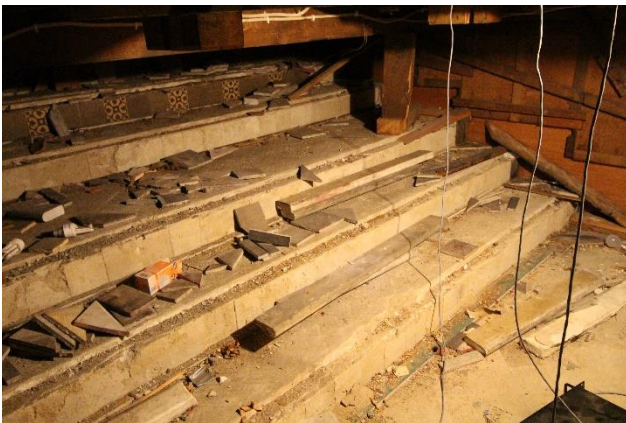
Figure 29 – Original stairs to Ark located under bimah.
