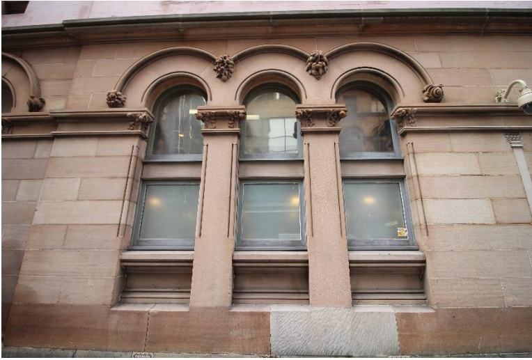
Figure 14 – Detail of ground floor windows with carved sandstone detailing.
