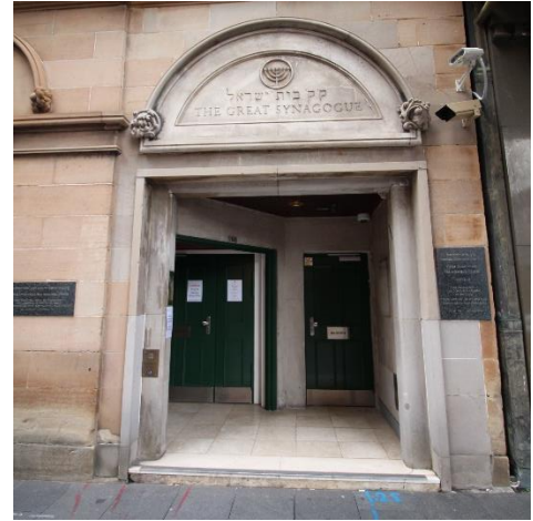
Figure 15 – Entrance at Castlereagh Street
