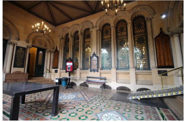
Figure 12– Elizabeth Street porch, west
