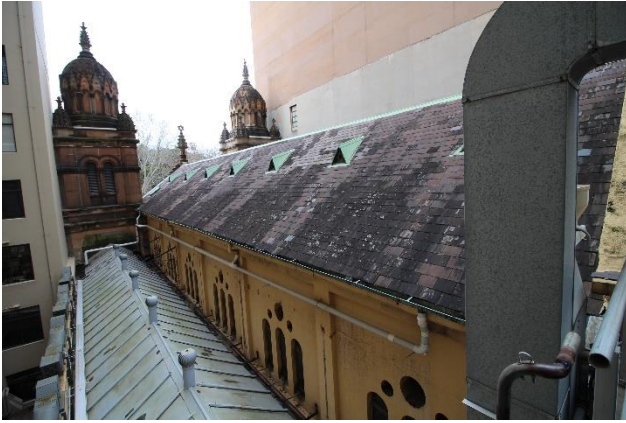
Figure 5 – Detail of roof.
