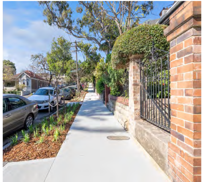
Images: Eglinton Road, Glebe Footway Renewal Works 2021
