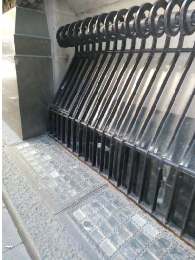
38 Original protective railing and glass pavement lights, Angel Place.
