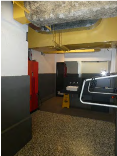
46 Original painted masonry structure evident in Bike Storage and Lockers Room
