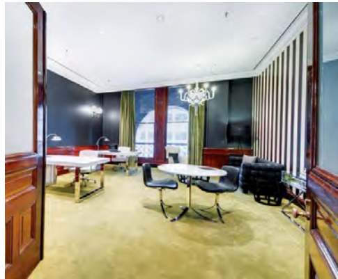
70 Office suite tenancy fit-out.
