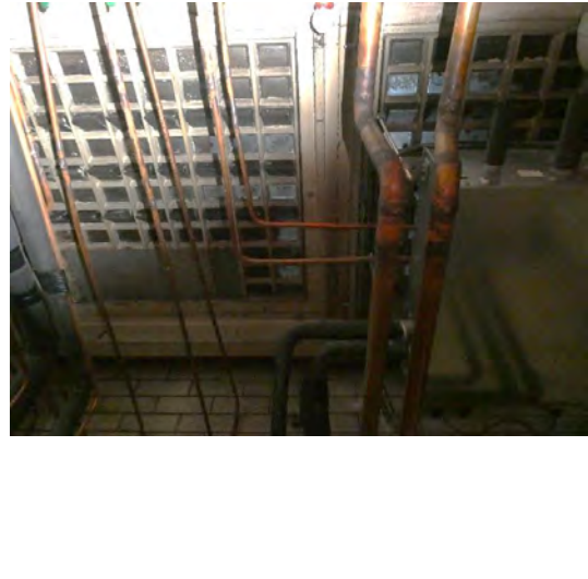
51 View to underside of original glass pavement lights on Angel Place.
