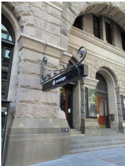
36 Non-original external scrollwork signage metal bracket with suspended signage attached to masonry stone piers on George Street.
