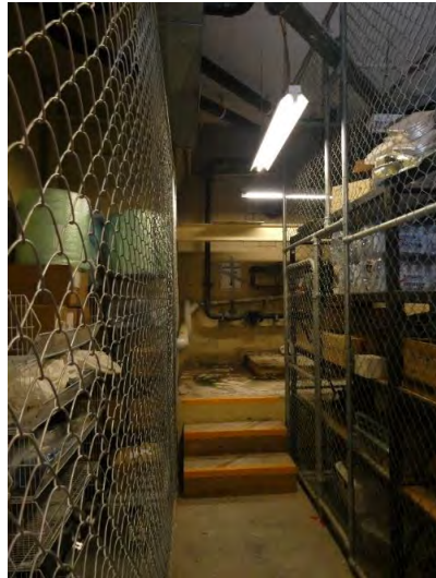
47 Temporary storage cages
