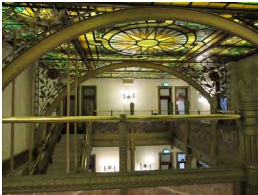
94 View to central atrium on the sixth floor. Reconstructed glass ceiling supported by two trusses.
