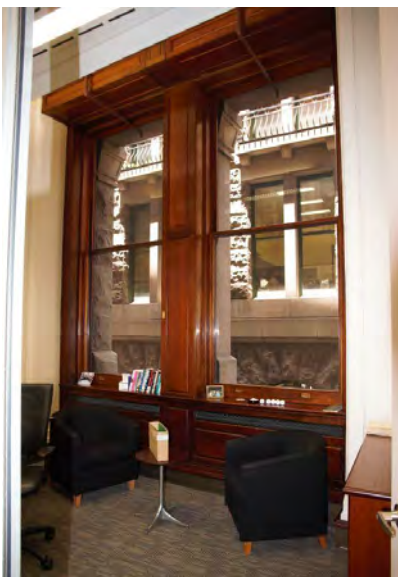
71 Original timber panelled windows.
