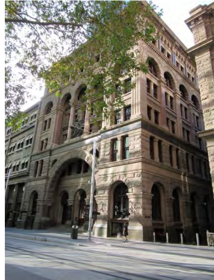
V2 Intersection of George Street, Angel Place, and Wynyard Street.
