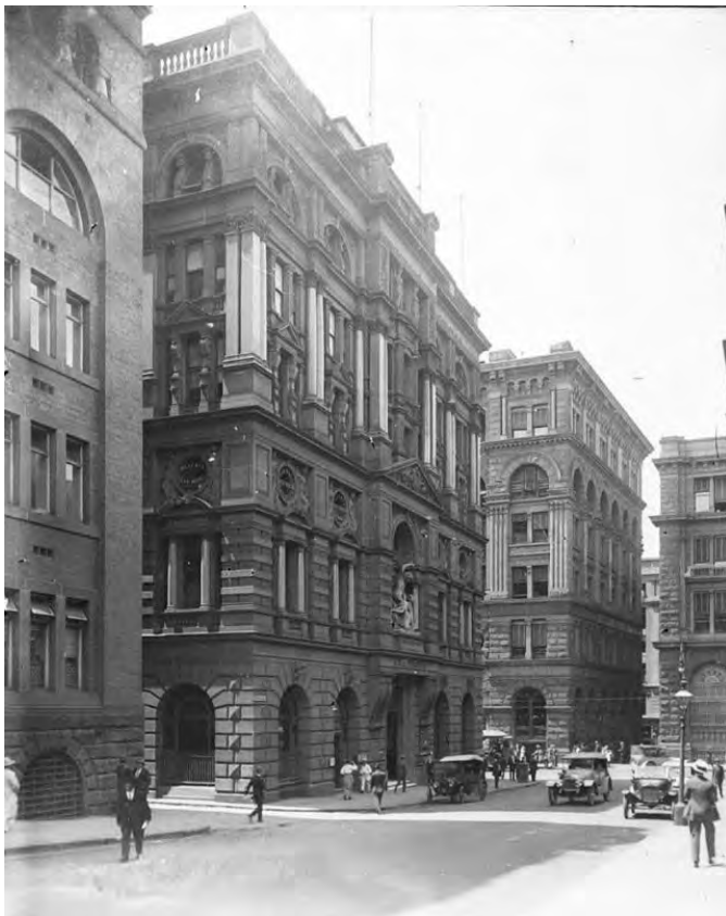
113 Looking east along Wynyard Street to George Street, circa 1915. Left to right: Lark Sons & Co warehouse (Jeaffreson Jackson, 1892-93); Mutual Life Association Building (John Sulman, 1890); Equitable Life Assurance Building of the United States (350 George Street, 1894) and Bank of Australasia (1904), both by Edward Raht.
