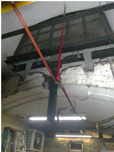
50 Original masonry structural arch.
