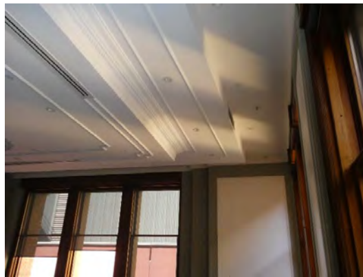
81 Detail of false ceiling, suite 309.
