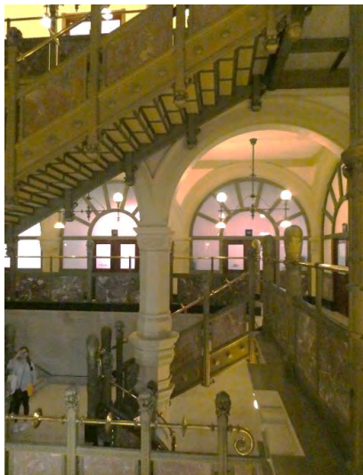
65 View towards north-eastern arcade.
