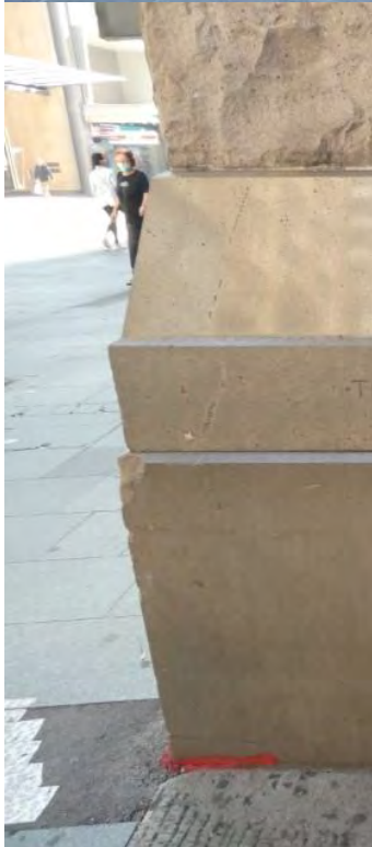
135 Damaged stone at the ground floor level of the Ash Street elevation (left) and at the south-western corner of the building. Repairs should be undertaken to the hydraulic system for the main entrance doors, located in the basement of the building, which is leaking.
