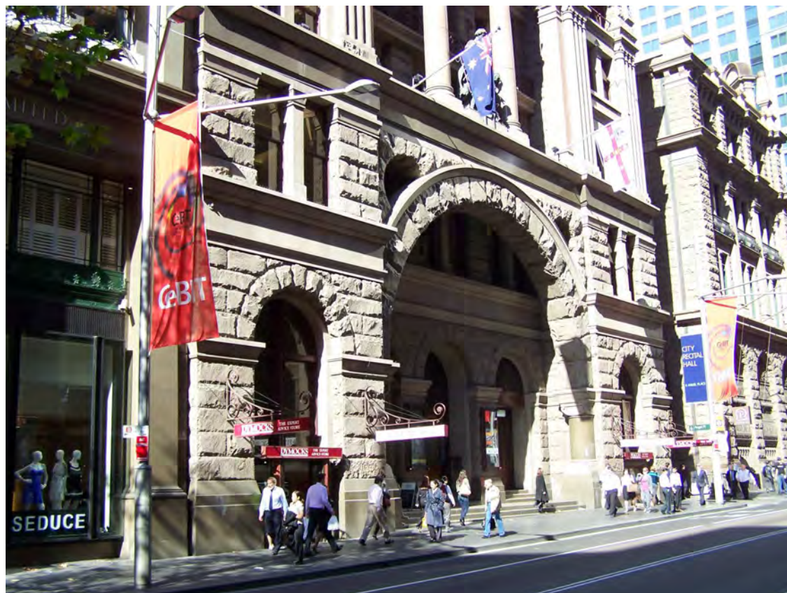
Figure 2 George Street façade at street level Source: Tanner Architects
