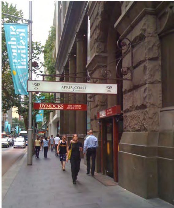
Figure 4 George Street façade at street level looking North
