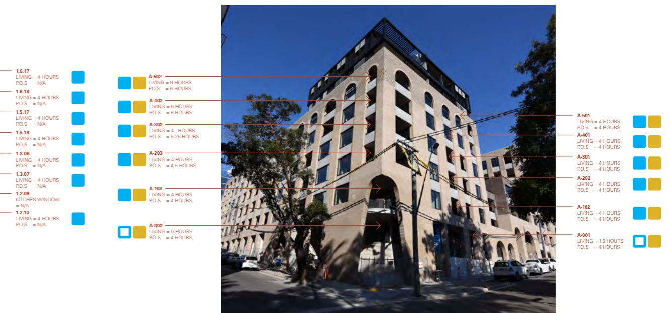
Existing - 14-26 Cowper Street
