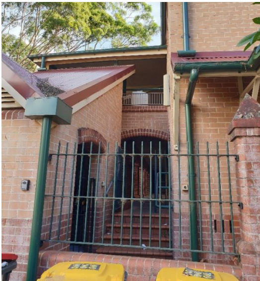
Figure 26. Stairwell at the north access to central courtyard of 17-31 Cowper Street, view looking south.
