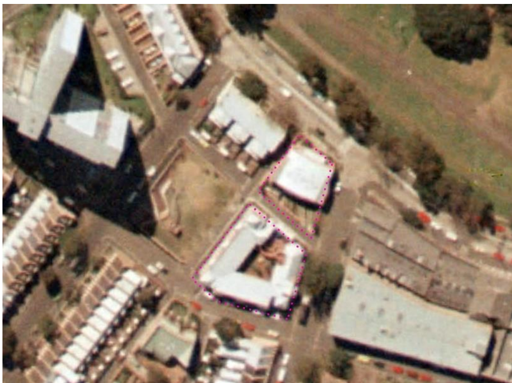
Figure 17. 1991 Aerial photograph with the site outlined in pink showing the two extant structures as they appear today. (Source: NSW Department of Finance and Spatial Services).
