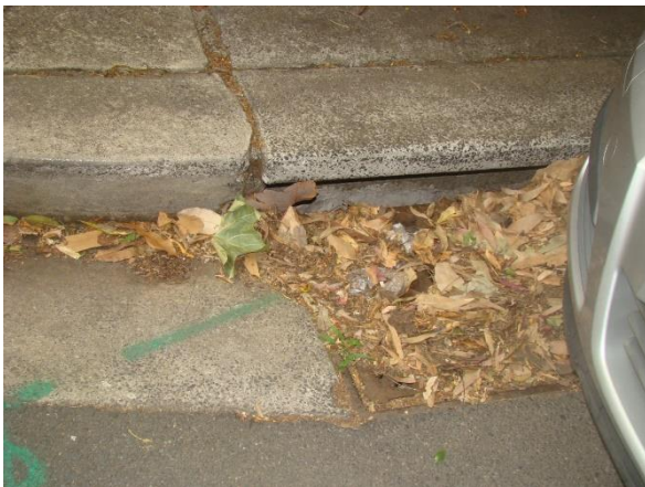
Figure 28. Street gutter inlet along Mitchel Line – obscured by dry foliage, looking east.
