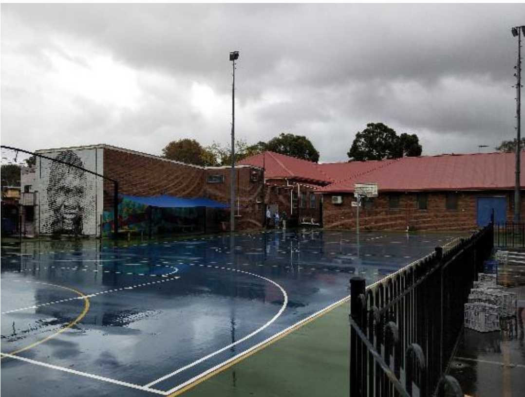
Figure 5. View of PCYC and basketball courts
