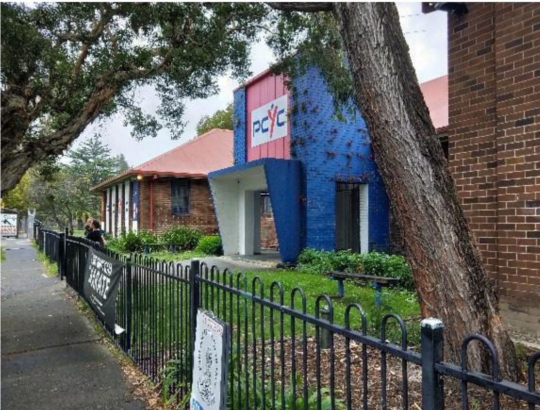
Figure 4. PCYC viewed from Elizabeth Street
