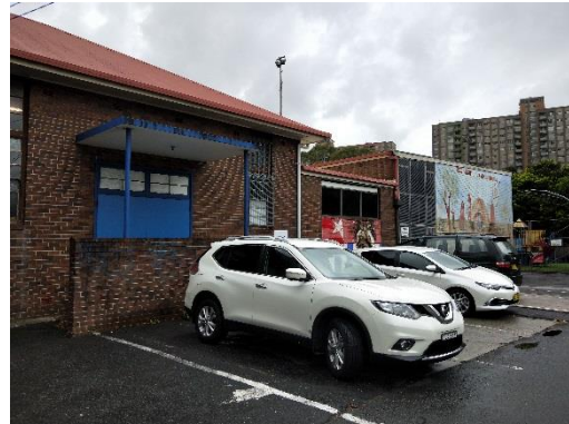
Figure 35 View of PCYC from Phillip Street
