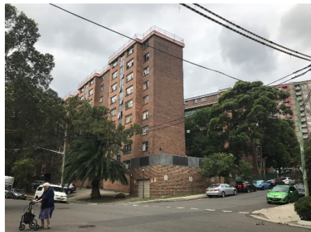
Existing 9-storey building on Kettle Street
