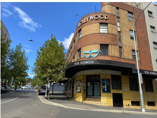
Figure 11: Hotel/pub opposite the site on Hunt Street
