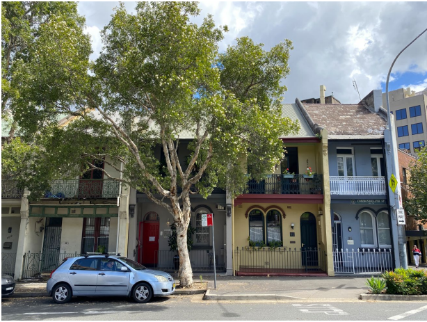
Figure 9: View of nearby terrace houses along Hunt Street
