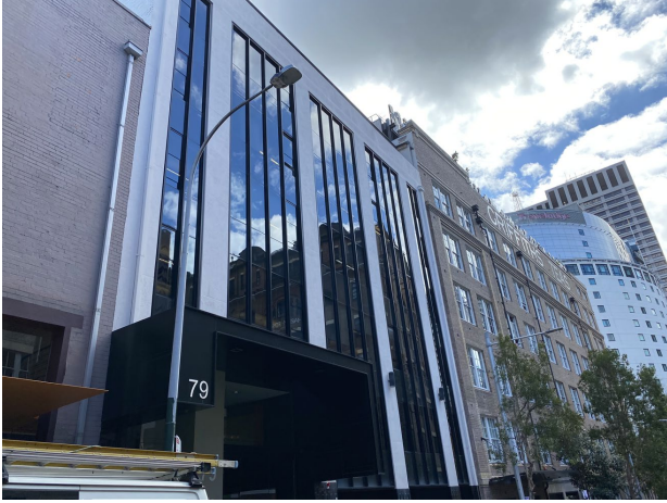
Figure 13: Commercial building adjacent to subject site - 79 Commonwealth Street (Commonwealth Street frontage)
