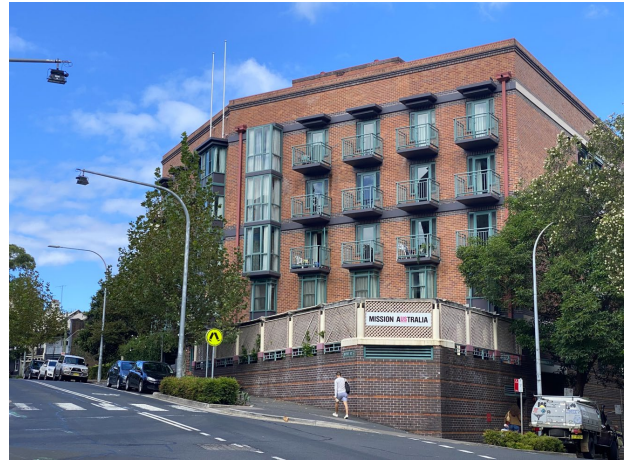
Figure 10: View of nearby multi residential building on Hunt Street
