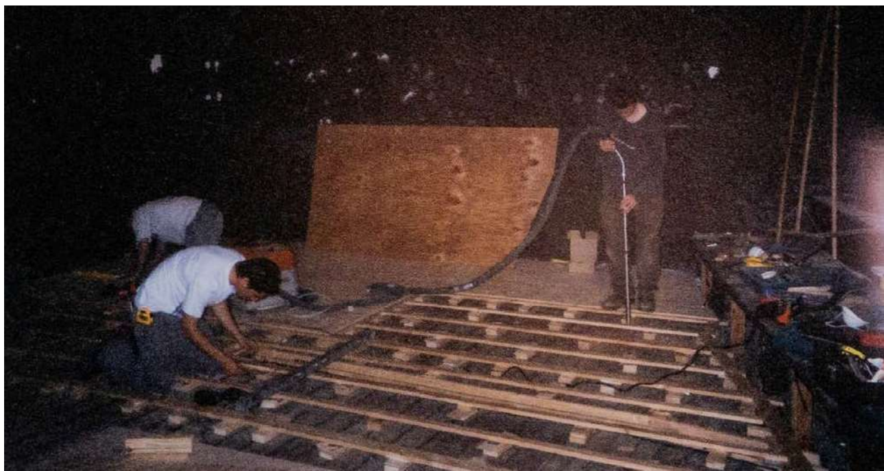
Figure 73: 2002. Stables Theatre Renovations. Source: SBW Foundation Archives.
