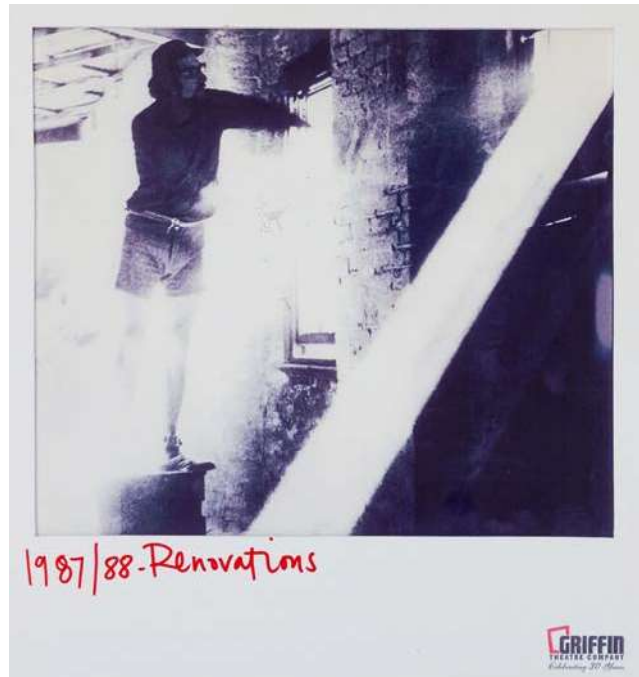
Figure 72: 1987-88. Stables Theatre Renovations. Source: SBW Foundation Archives.
