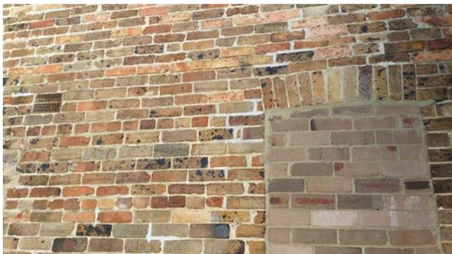
Figure 107: Brick infilled windows and different designs of metal ventilation grilles found on main facade facing Nimrod Street.
