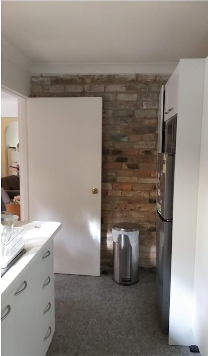
Figure 155: Exposed face brick wall defining kitchen.
