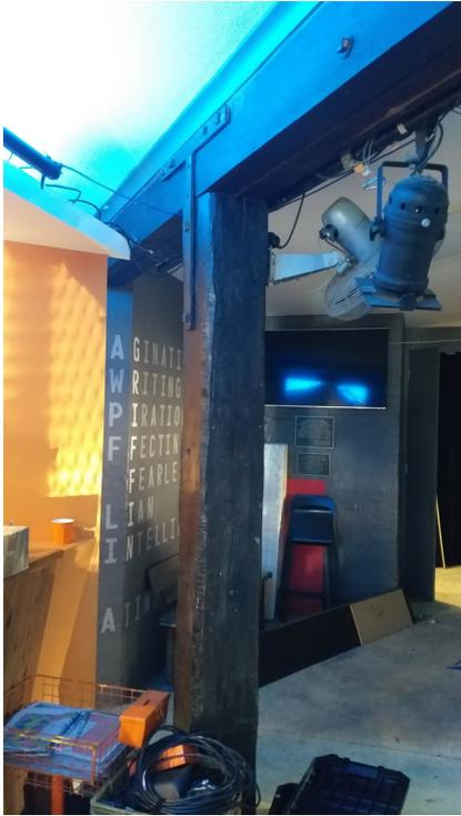
Figure 121: View of timber column and beam supporting the upper levels and separates the foyer and bar areas.
