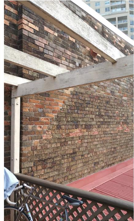
Figure 157: View of brick repairs to external wall of SBW Stables Theatre. Roof over kitchen visible.
