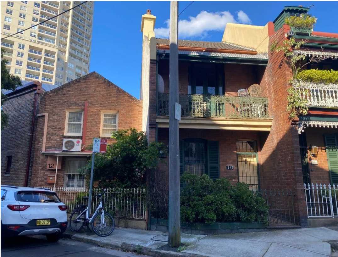
Figure 6. 12 Nimrod Street and adjoining development to the south-east, viewed from south-west
