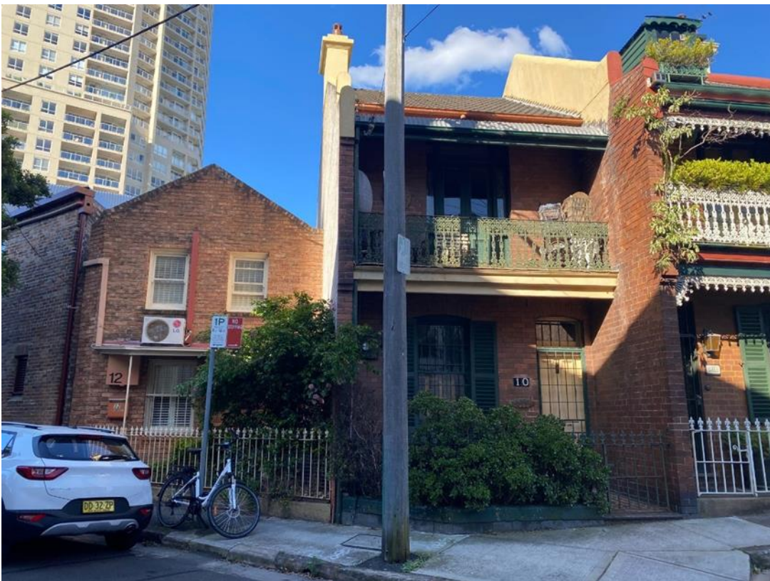
Figure 6: 12 Nimrod Street and adjoining development to the south-east, viewed from the south-west
