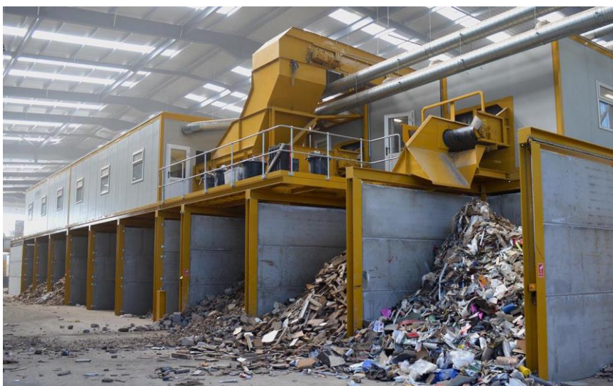
Figure 17: Construction & demolition waste recycling facility
