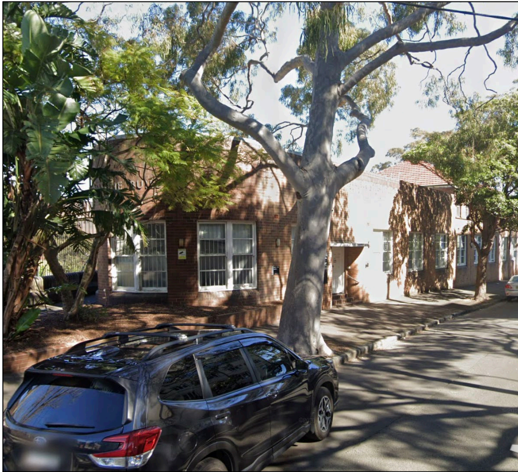
Mackie Building, 2 Arundel Street, looking west
