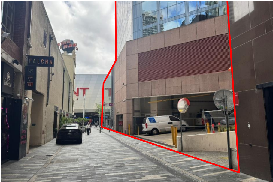
Figure 8. Looking west along Wilmot Street with the subject site (in red) on the left
