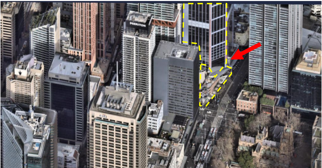
Figure 36 View of the Sydney CBD looking south toward the subject site – marked by red arrow (yellow dash highlights the subject tower and podium).
