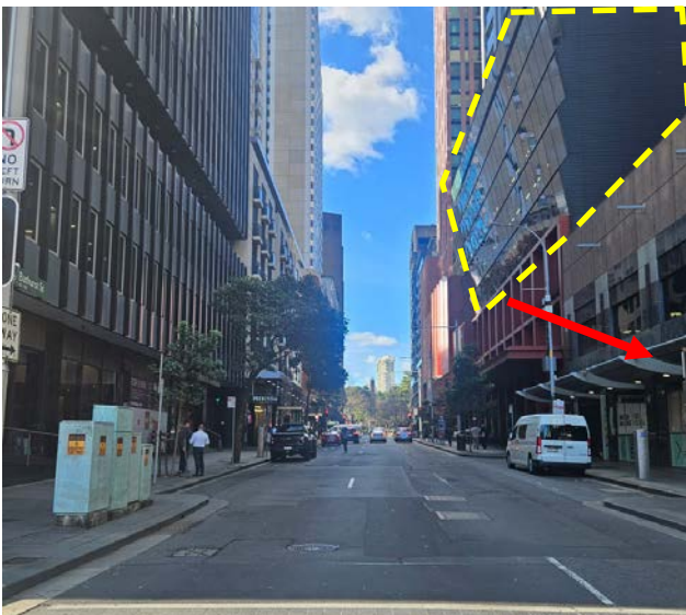
Figure 39 View looking east along Bathurst Street, subject site marked by red arrow and the adjacent building shown in yellow dash. The PP envelope aligns with the height of this adjoining development
