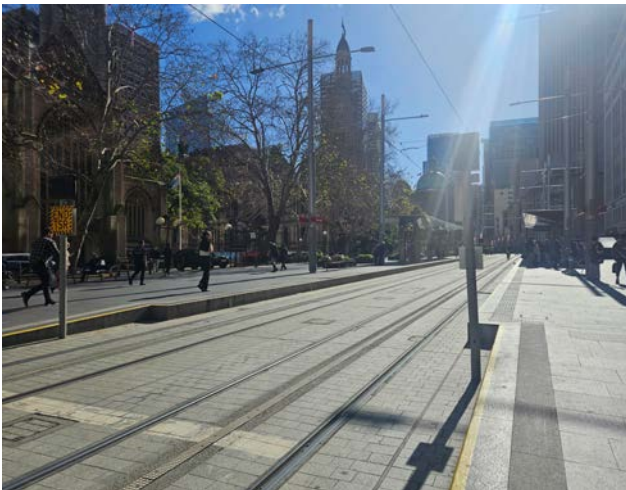
Figure 4 View looking north along George Street towards the Town Hall and the Cathedral and showing the light rail infrastructure
