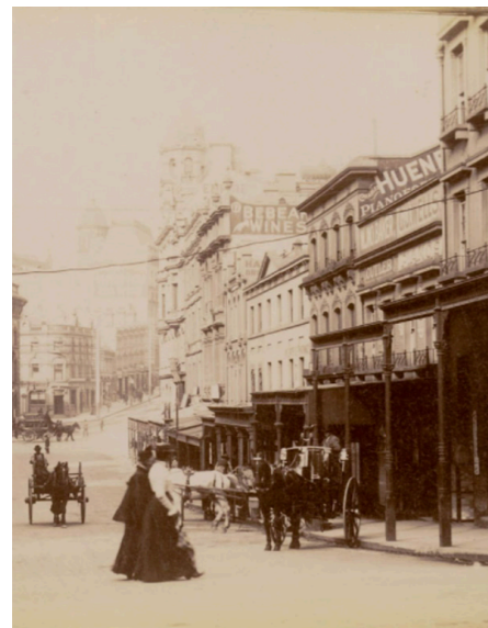
29. View looking East from George st along Hunter st, 1900-1910. Former Skinner's Family Hotel to the right of image. Subject Western Metro site is situated.
