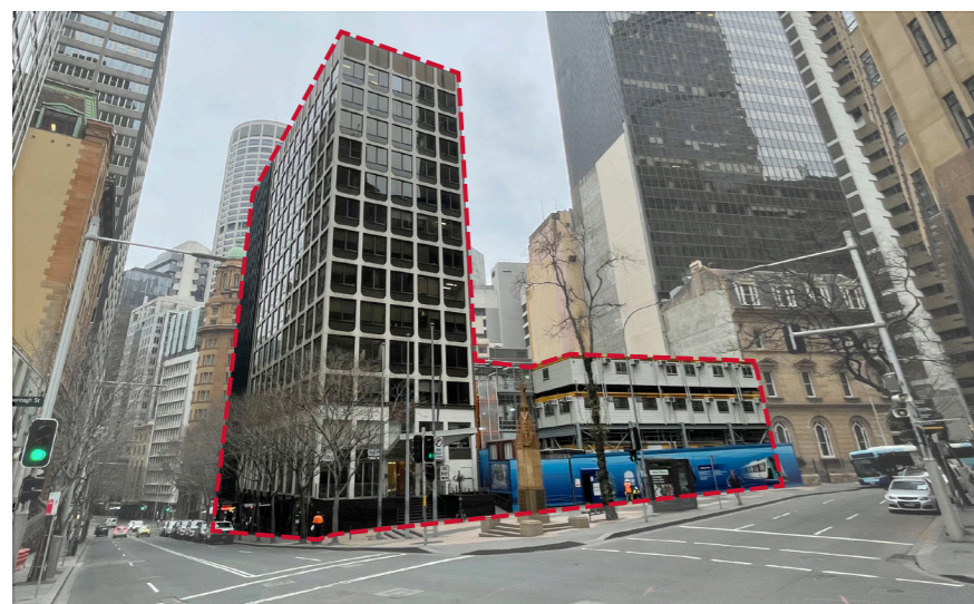
18. Existing Development - Hunter Street East
