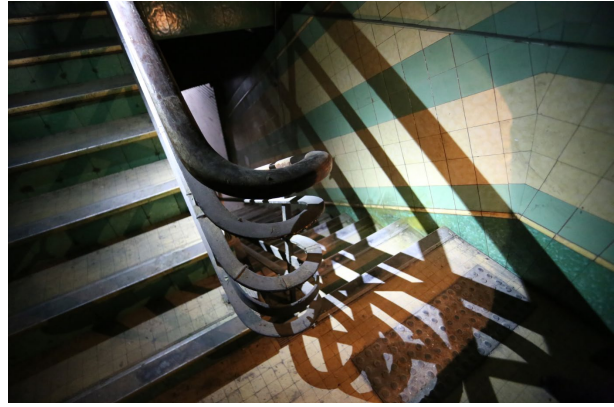
Figure 75 – Timber and iron balustrade
