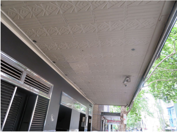
Figure 10 – Pressed metal ceiling
