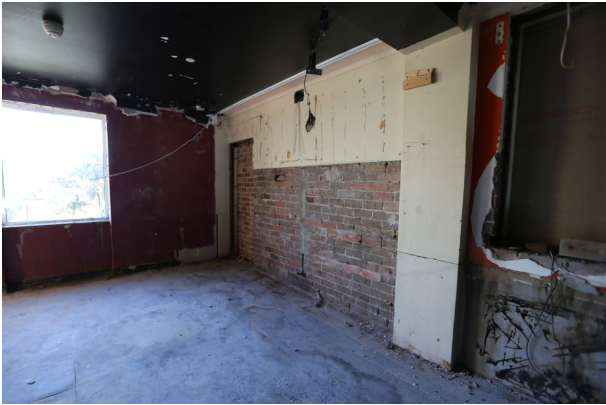
Figure 77 – View of the north-west corner of the bar area. Former door opening has been infilled on the left end of the wall.
