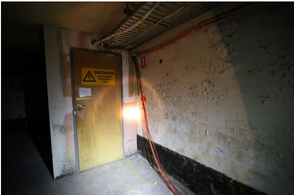
Figure 39 – Switch room with lightweight partition walls. Located in the south-east corner.
