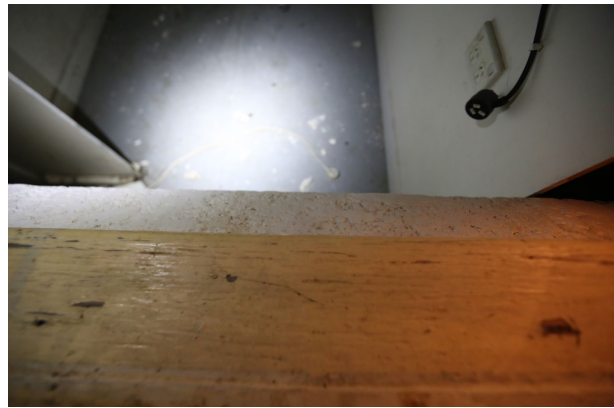
Figure 98 – Evidence of the formerly exterior wall and windowsill (remnant of lightwell).
