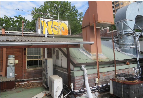
Figure 25 – View of the former skylight (now used for mechanical ventilation). The top of the southern parapet can also be seen through the service vents.
