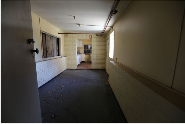
Figure 114 – View west into a later infill between an original small laundry room. The original external brick walls can be seen with lightweight walls placed above.
