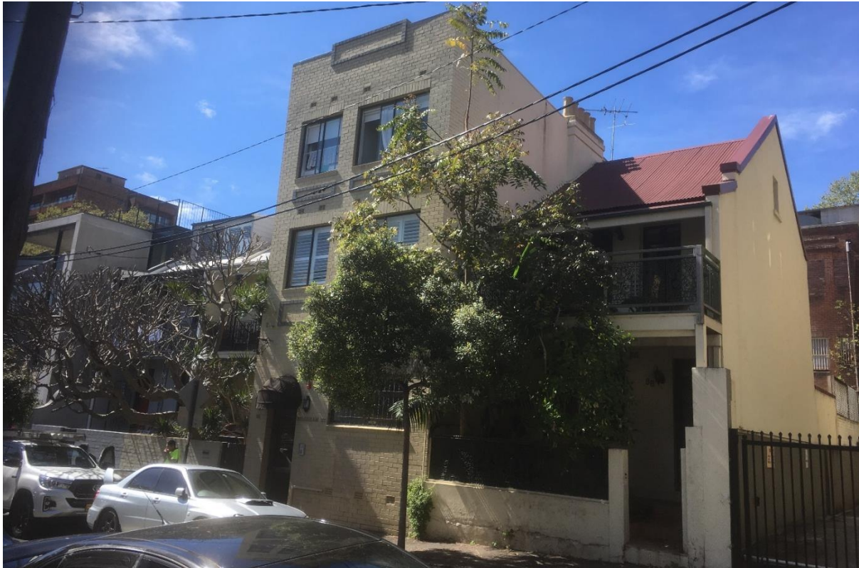
Figure 4: View looking east to the planning proposal site showing three terrace dwellings and a residential flat building at 92-98 Brougham Street
