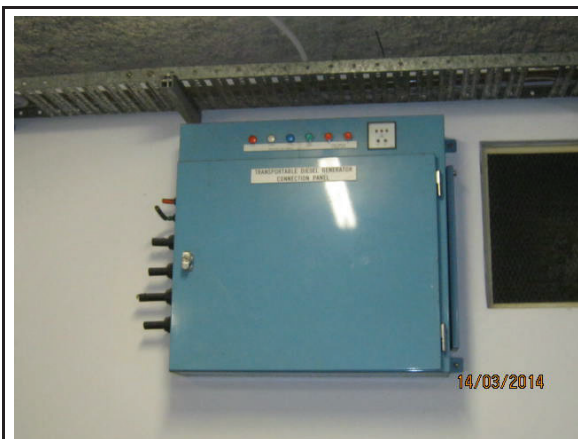
Photo 9: Disconnected power box to diesel AST
