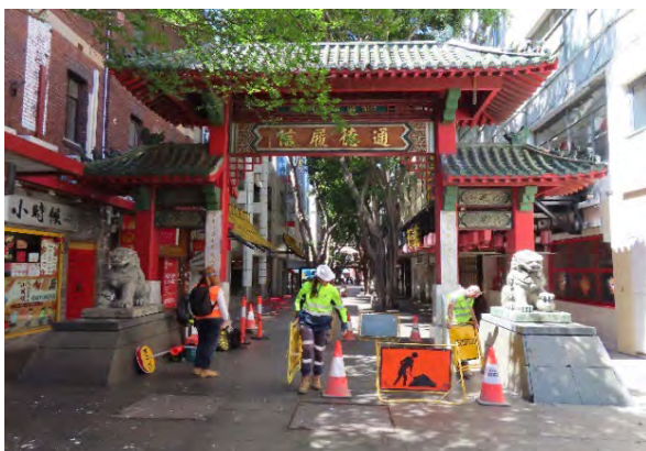
Figure 4.2 North elevation (image taken from the north).
