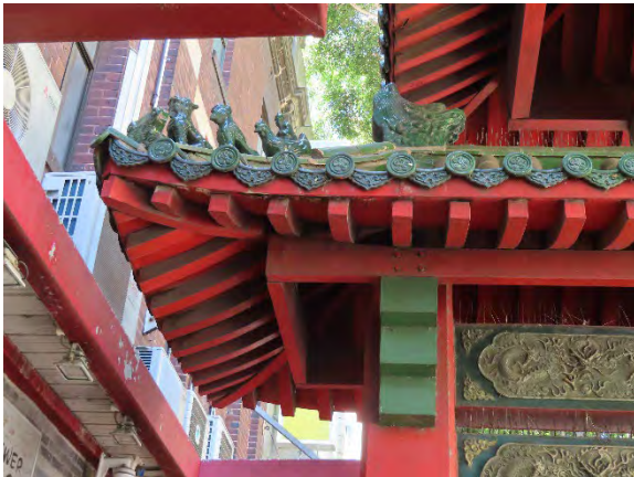
Figure 4.14 Symbolic ceramic capping tile figures on the hip of the lower roof—eastern bay.
