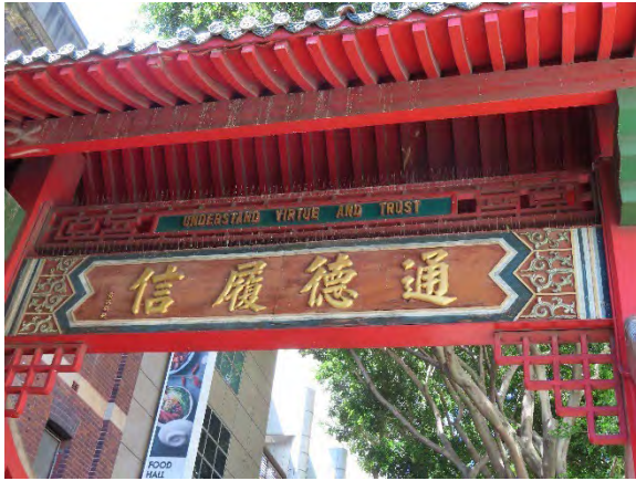
Figure 4.4 Panels A and B on north elevation with inscription in English above and Chinese below: 'Understand virtue and trust'. Decorative lattice brace C beneath panel B.
