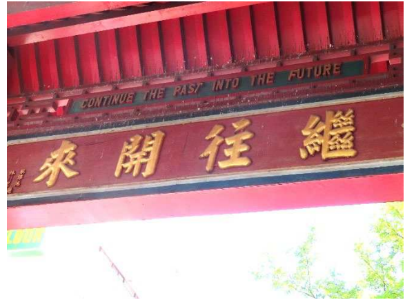
Figure 4.5 Panels A and B on south elevation with inscription in English above and Chinese below: 'Continue the past into the future'.
