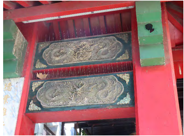
Figure 4.9 Decorative moulded panels E and E' featuring motifs in fibreglass at the western bay.
