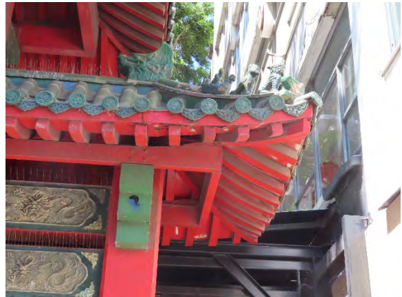
Figure 4.15 Symbolic ceramic capping tile figures on the hip of the lower—western bay.
