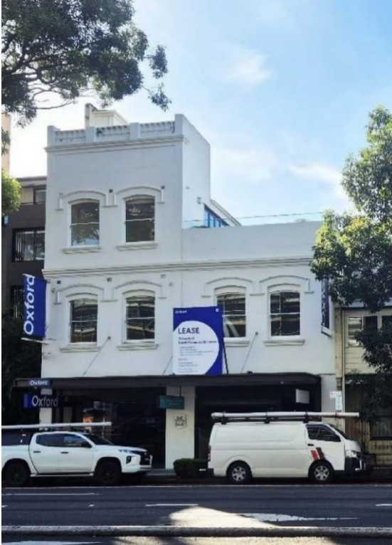
Figure 5. 40-42 Flinders Street, Darlinghurst. Photo: TKD Architects
