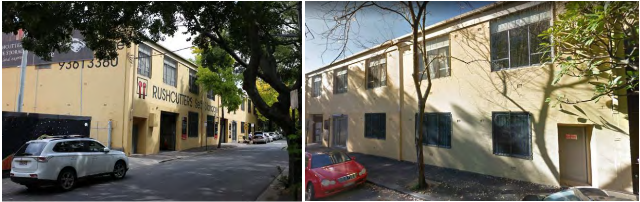
30-62 Barcom Avenue, looking south
