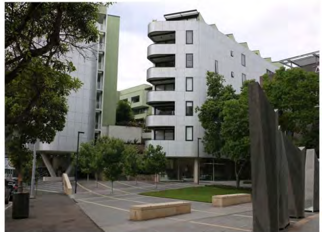
View of mixed use development, plaza and commercial showroom at McLachlan Avenue, looking east
