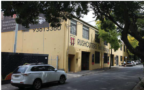
11 View 1 - Looking south at the Site's primary frontage
