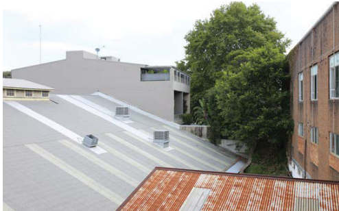
19 View 3 - Looking towards the residential interface to the rear of the Site
