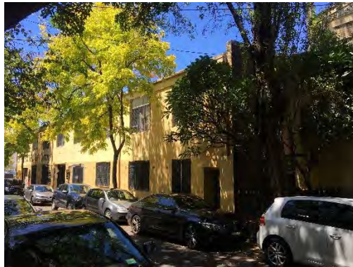
Figure 22 – View of the existing face brick building as seen along Barcom Avenue.
