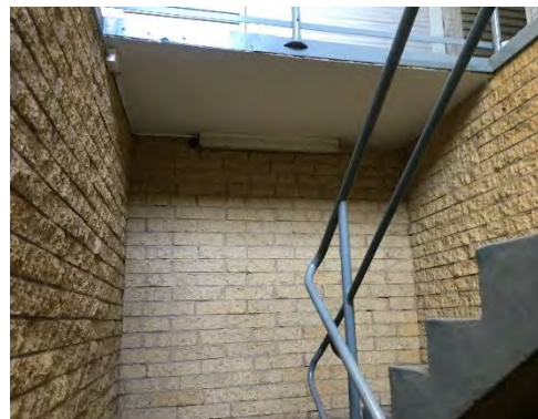
Figure 25 – Finishes as seen at the staircase leading up to the first floor.
