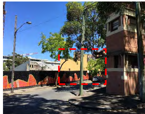
Figure 10 – View from the corner of Womerah Avenue and Barcom Avenue looking southwest towards the subject site outlined in red. 65 Craigend Street is located immediately to the north.
