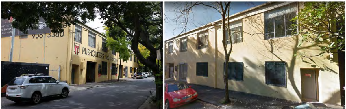
Figure 3: Photographs of the site and existing building, (L-R) looking south and looking north-east
