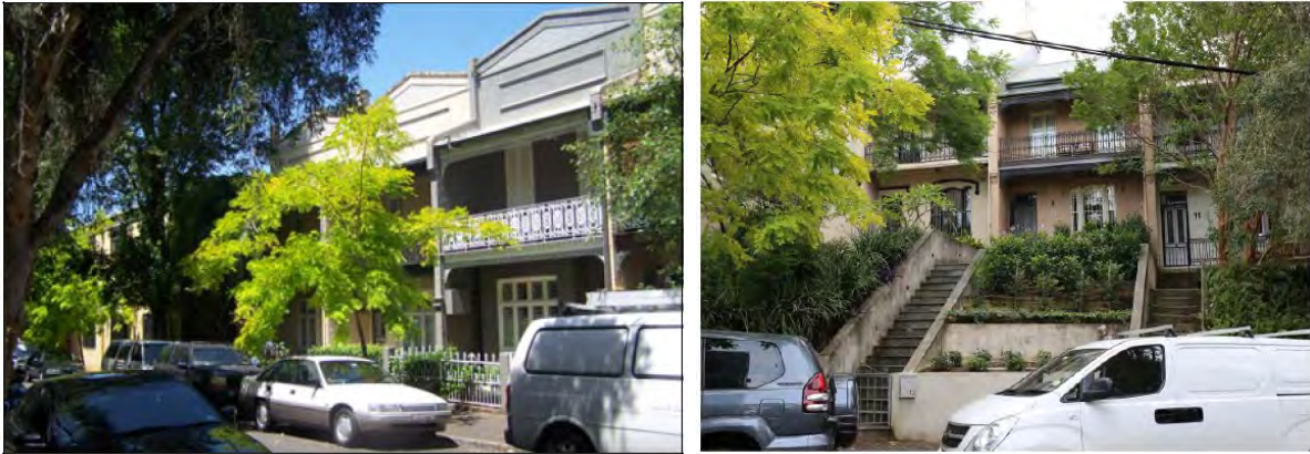
Figure 4: Adjoining residential terraces, (L-R) to immediate south of site along Barcom Ave and heritage items on the opposite side of Barcom Ave within the conservation area
