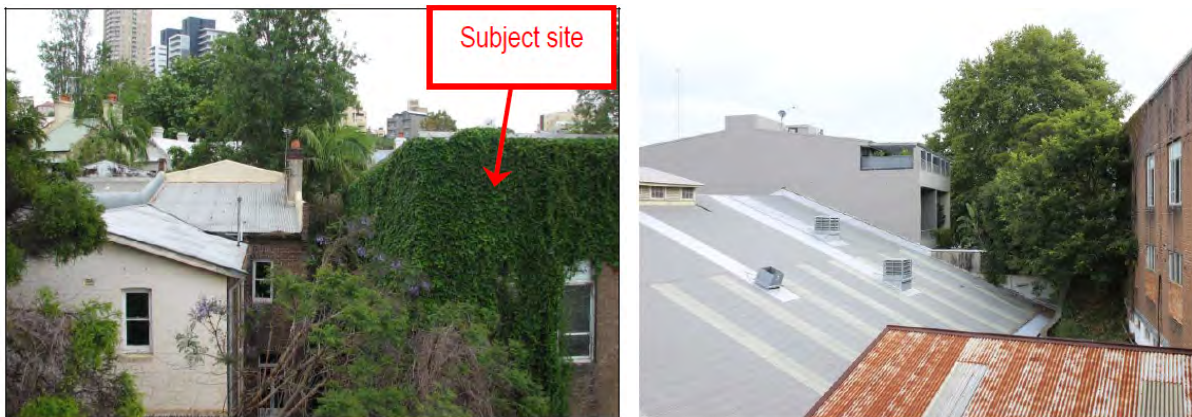
Figure 5: Residential interface with site, (L-R) 2 storey terraces to south-east of site and view towards four storey residential building to south of site
