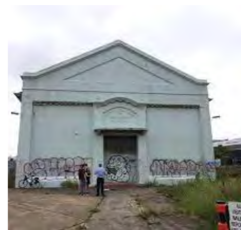
Sydney Water Valve House
