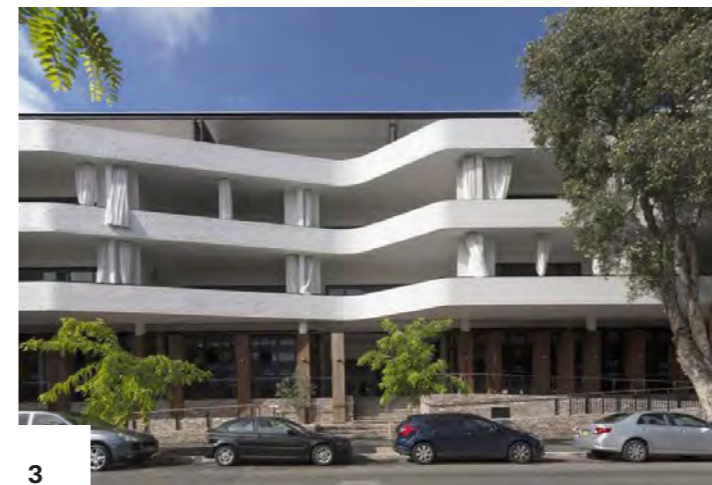
3 Casba, Danks Street
