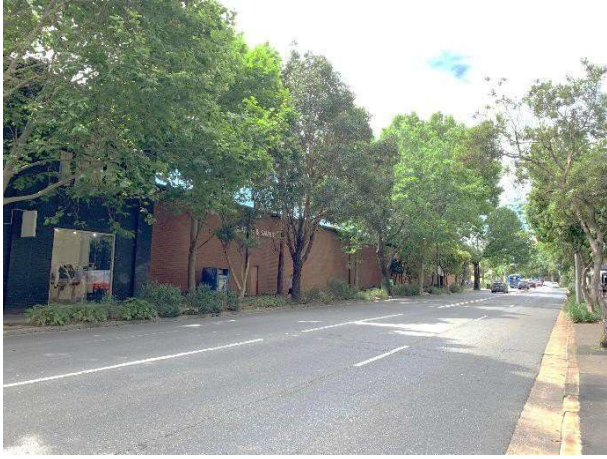
View looking north on Bourke Street along frontage of site
