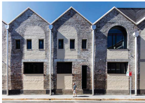
① Old - New Brick Facade Juanita Nielsen Community Centre, Woolloomooloo NSW (Neeson Murcutt Architects)
