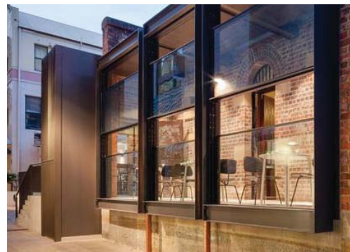
③ Mild steel with micaceous iron-oxide paint finish Former Rocks Police Station, The Rocks NSW (Welsh+Major)
