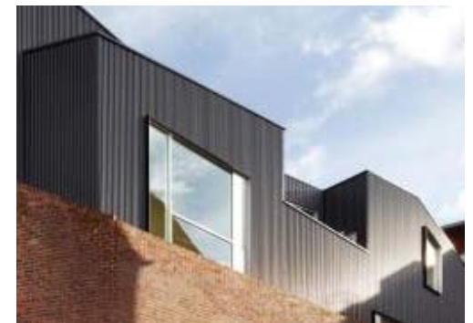
④ Powder coated aluminium profiled sheet cladding 192 Shoreham Street, Sheffield UK (Project Orange)
