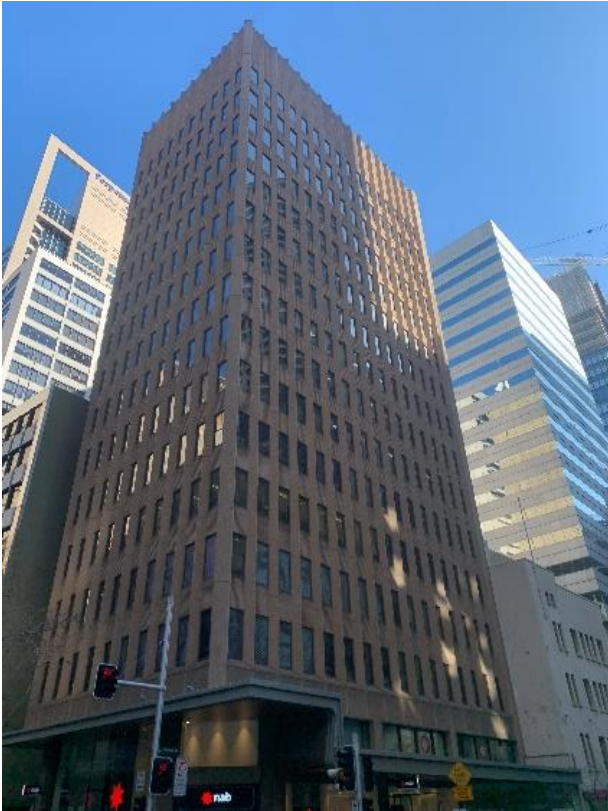
Figure 25 Currency House at 23-25 Hunter Street
