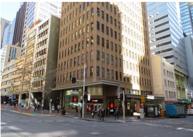
Figure 33 The subject site at the southwest corner of Pitt and Hunter Streets
