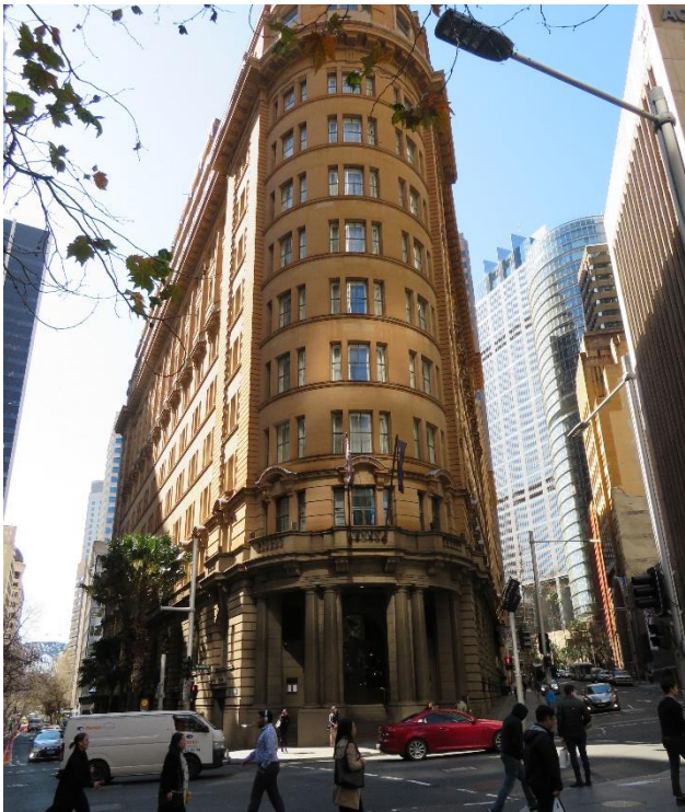
Figure 39 View east along Hunter Street, towards the heritage listed Former Wales House at the intersection
