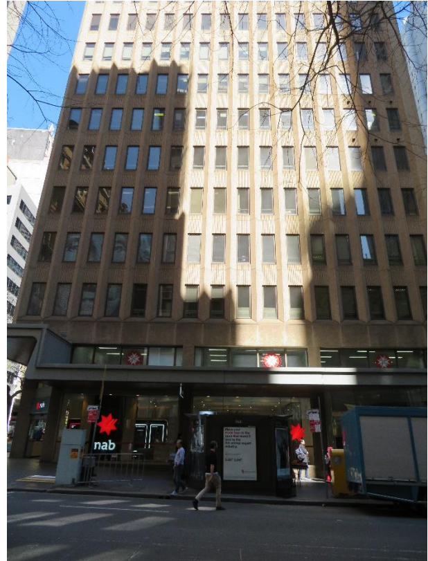
Figure 26 Currency House (northern Hunter Street façade)
