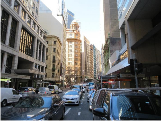
Figure 37 View east along Hunter Street, towards the heritage listed Former Wales House at the intersection
