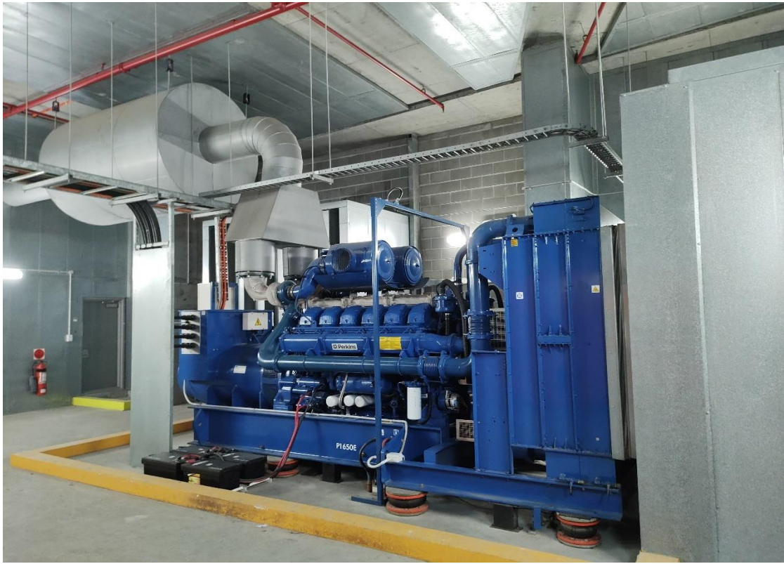
Photo 11: Diesel generator room in level 7
