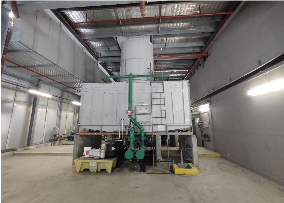
Photo 5: Coolin tower room in level 19
