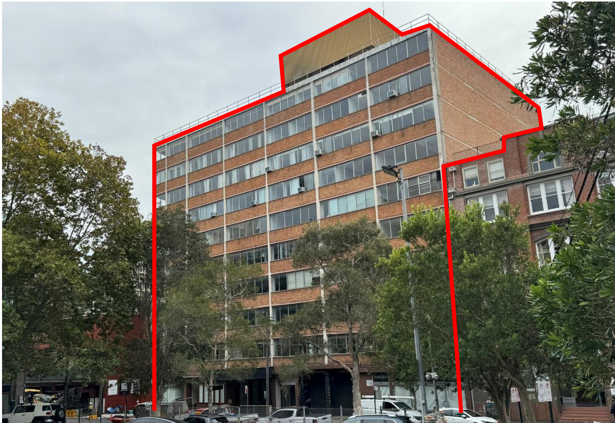
Figure 2: 8-24 Kippax Street, viewed from the south-east outlined in red
