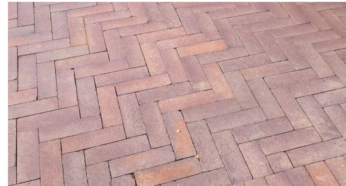
Example of new brick paving
