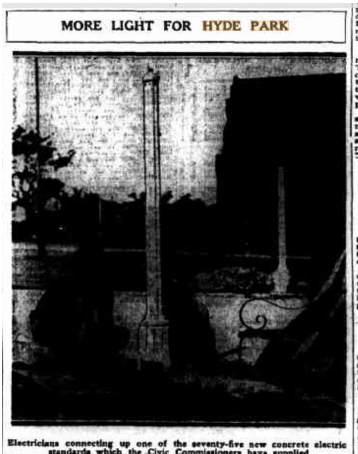
Figure 5.4 One of the concrete lighting standards being installed in Hyde Park. (Source: The Labour Daily 6 November 1929)
